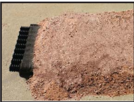
Cover with clean, very coarse sand before bringing in fill.
